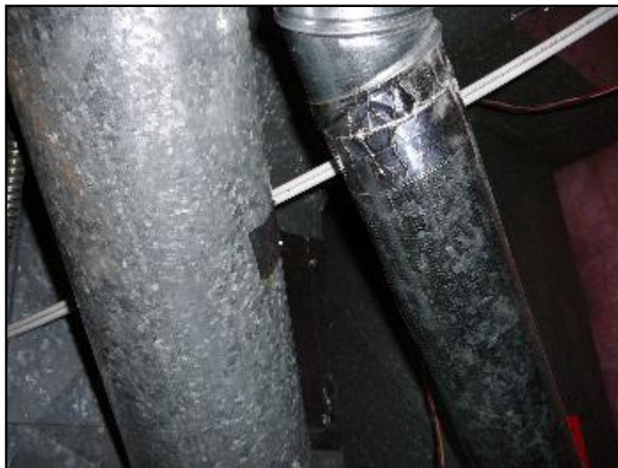
move wire - provide proper support
