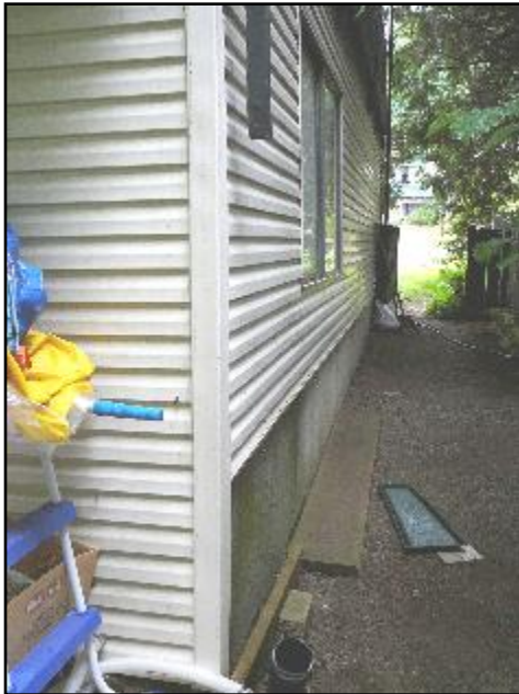
add downpipe to connect to drain
