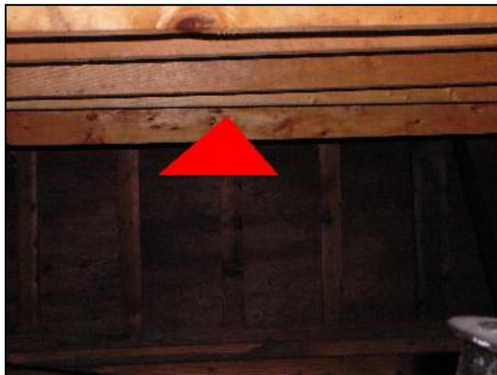
repair collar tie
